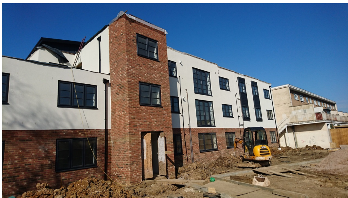
New homes being built at former Twin Foxes site
